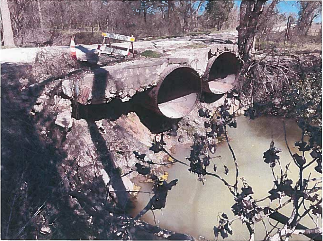
View from Upstream
